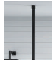
Close up of vertical ceiling support bar
